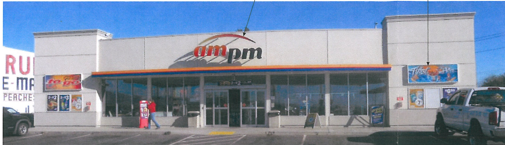
PHOTO OF EXISTING BUILDING ON SITE
